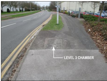
PHOTOGRAPH 4 EXISTING LEVEL 3 CHAMBER IN FOOTWAY ON DONCASTLE ROAD OUTSIDE BUILDING
