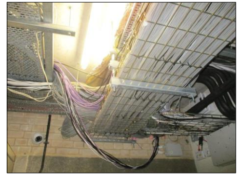
PHOTOGRAPH 12 TYPICAL VIEW OF OUTGOING TELECOMS SERVICES TO RISER AT HIGH LEVEL IN TELECOMS ROOM
